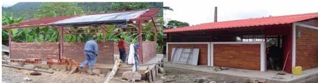
Photograph 3: Advances of the construction
