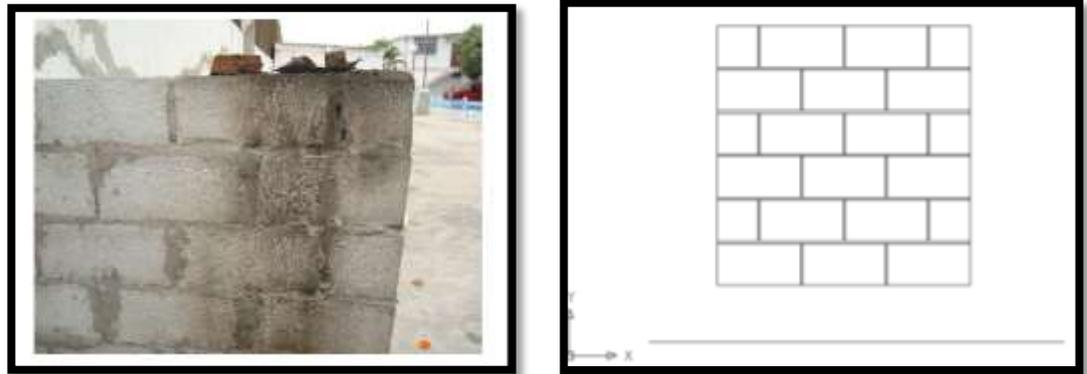
Figura 4-4: Pared incinerada
