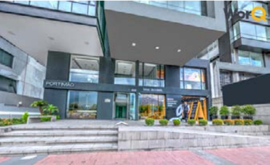
Figura 38. Fachada “Coworking WorQ”
