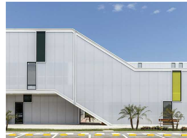
FIG 62. Hospital general de Manta, PMMT, Ecuador.
