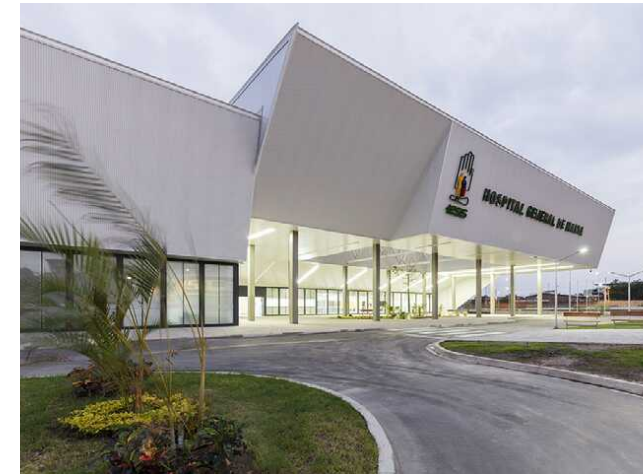
FIG 61. Hospital general de Manta, PMMT, Ecuador.
