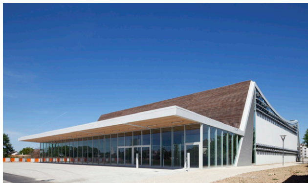
Paneles Brise- soleil
