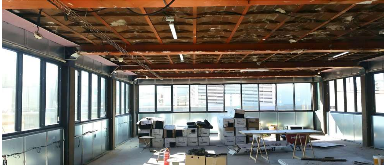
Interior paneles sin emplacar COAC
