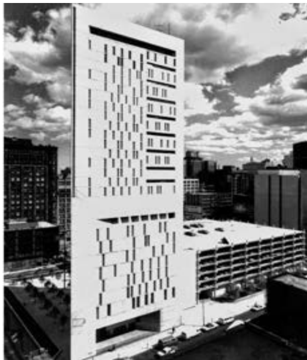
Fig. 08. Metropolitan Correctional Center, 1975 Fuente: Jonathan Choe
