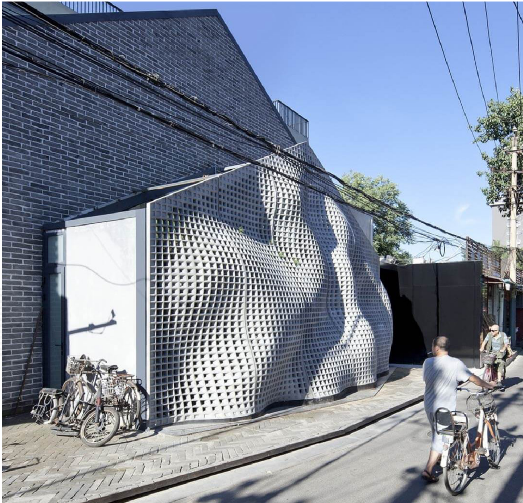
Figura 7: Exterior "Mao house"
