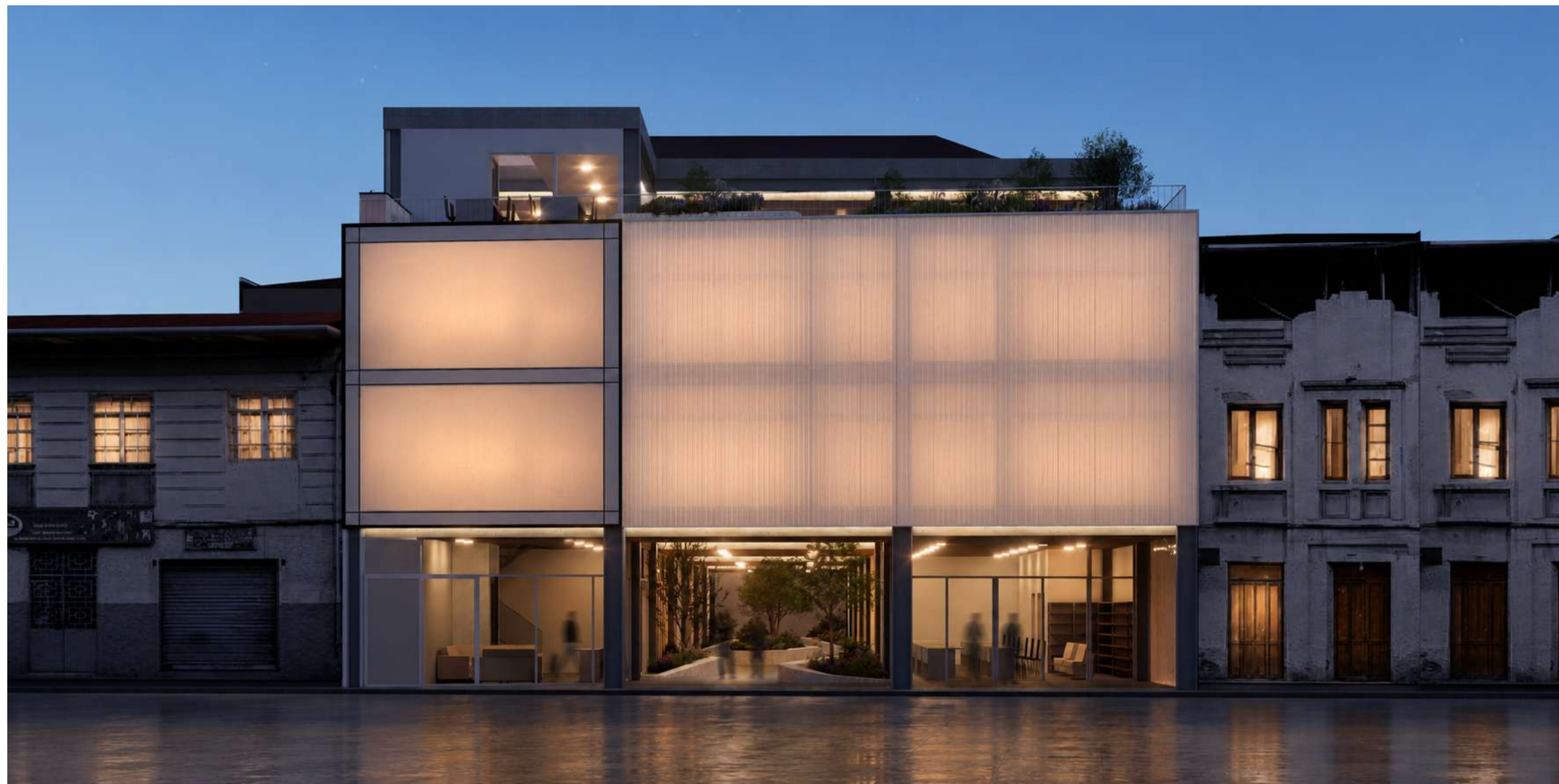
FACHADA MARISCAL LAMAR
