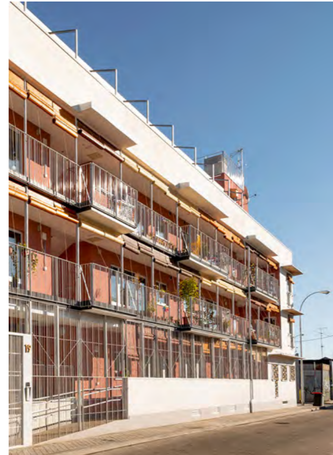
Fig. 16 Fachada Cohousing Entrepatios
