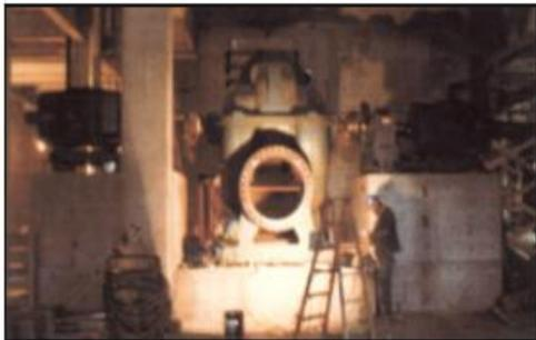
Disassembled pump prior to installation
