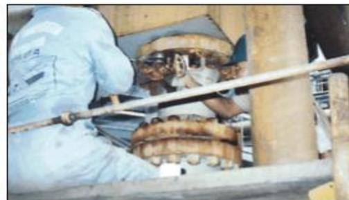
*Previously, 3 men with hot work permits were required for 6 hours to disassemble flange bolts.*
