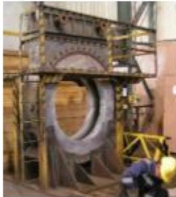
On top of the valve is a rectangular tongue and groove flange. In the past the customer used asbestos packings next glass, graphite, ceramic ropes. Due to thermocycling, incorrect assembly without torque wrench, wrong bolts and sealing materials this flange failed frequently.
